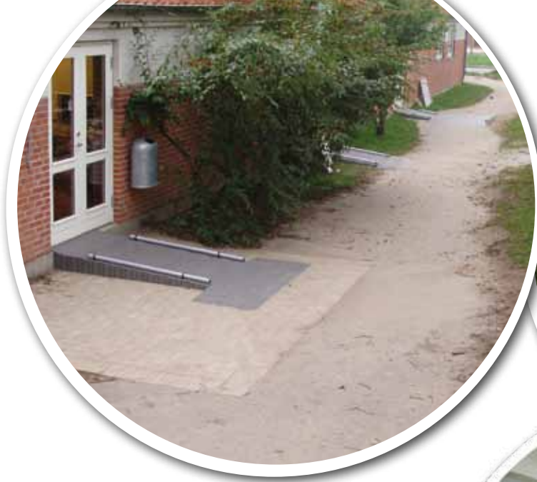
Three kindergarten ramp installations.
