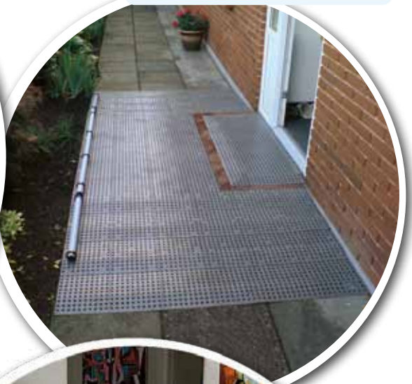
Ramp built around a platform. Note the corners of the platform.
